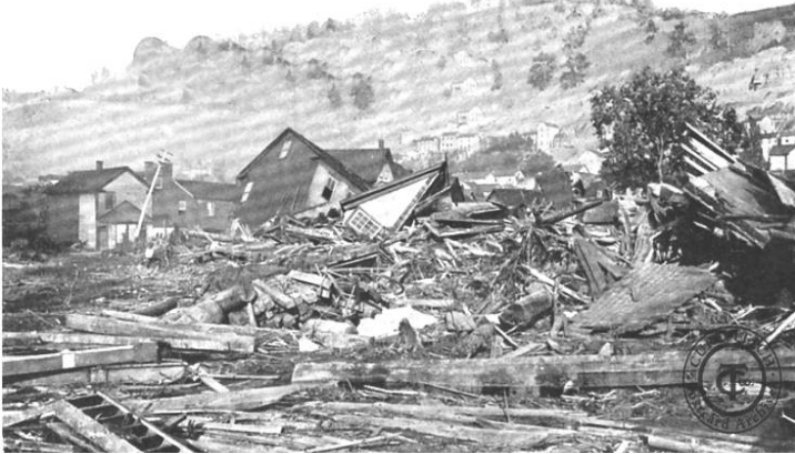
Houses Crushed by the Powerful Waters, Johnstown Flood, May 31st, 1889, Johnstown, Pa.
